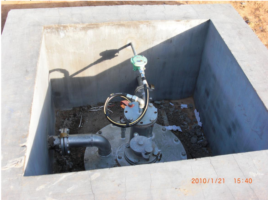
After Level gauge installation
