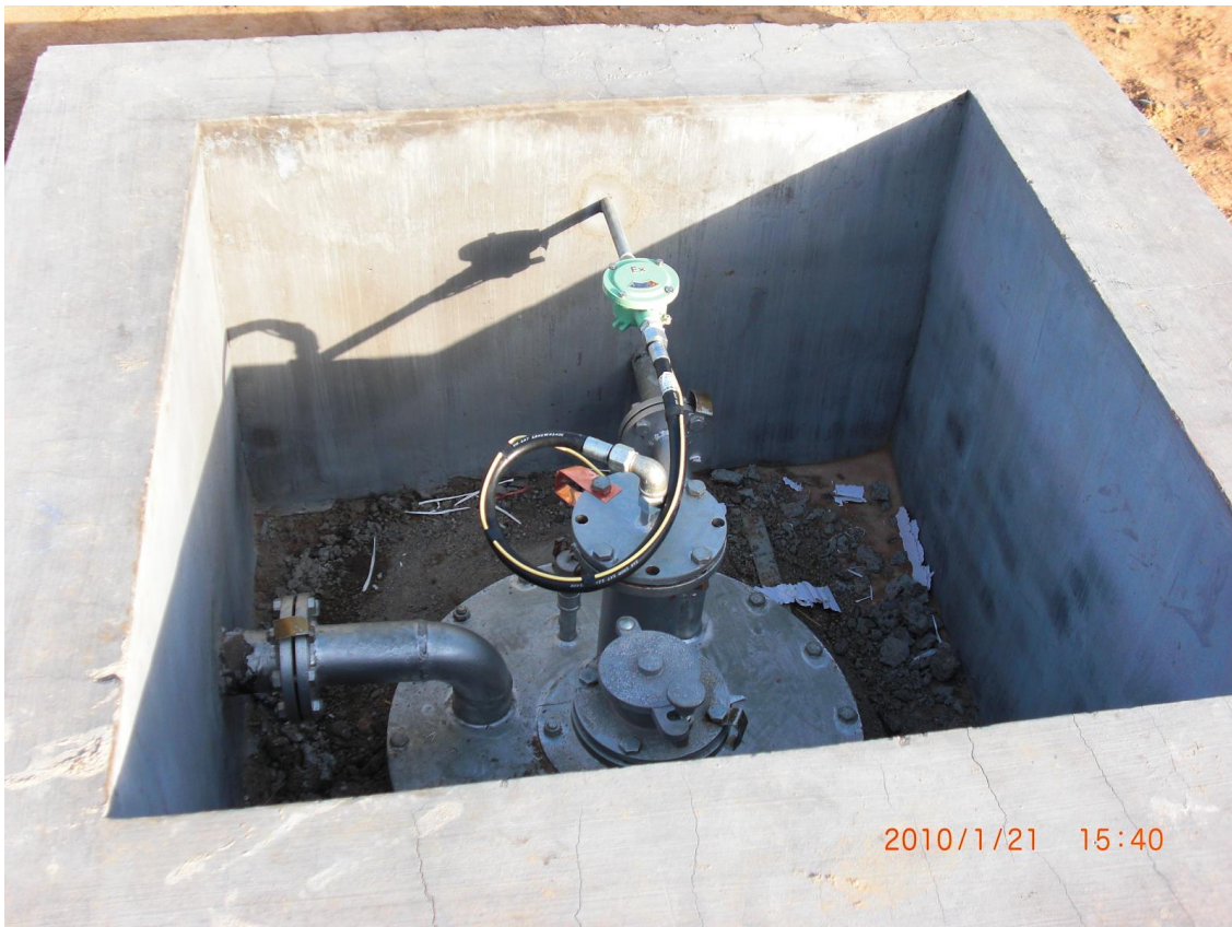
After level meter installation
